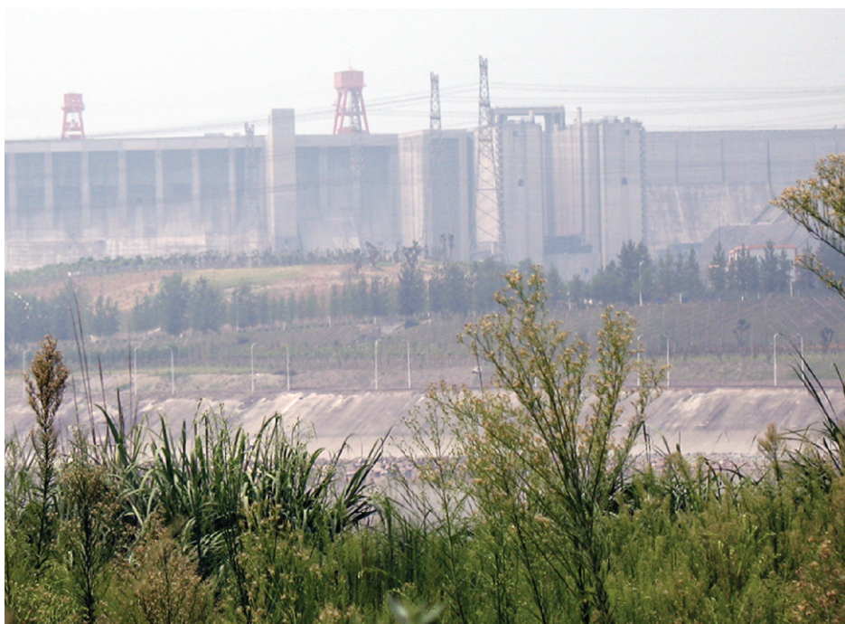
Figure 5. An invasive plant, broadleaf fleabane ( Conyza sumatrensis ), now dominates the flanks of tributaries near the Three Gorges Dam. Disturbance caused by dam construction has provided much new habitat for this plant invader. Photograph: Jialiang Zhang.
