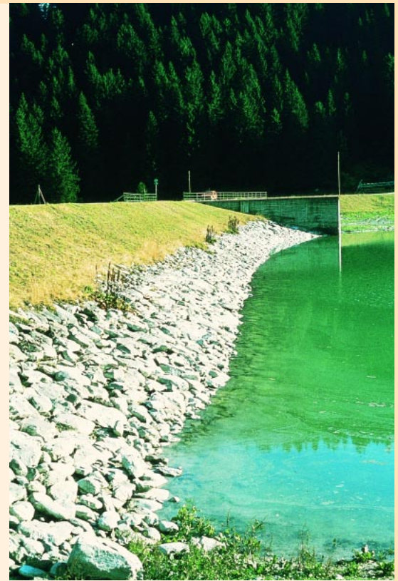
FIGURE 7 Environmental improvement for hydropower production and operation: This highly artificial shoreline at a small-scale hydropower reservoir near Brigels in eastern Switzerland (Rhine Valley) illustrates the potential for ecological improvement of many hydropower plants. Revitalizing surface waters could both improve habitat quality for aquatic forms of life and enhance aesthetic appeal to tourists. (Photo by B. Wehrli)
