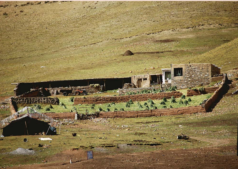
28 FIGURE 2 The “Four-Way Scheme” policy: a winter house, livestock shelter, fence (wall), and winter fodder are shown here, along with a traditional tent in the foreground. (Photo by author)
