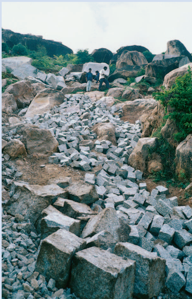
FIGURE 5 Stones being prepared for use in construction. This valuable source of income unfortunately leads to depletion of the very resource on which it relies; excessive stonecutting also degrades the environment, causing erosion and loss of topsoil. (Photo courtesy of Sampark)
