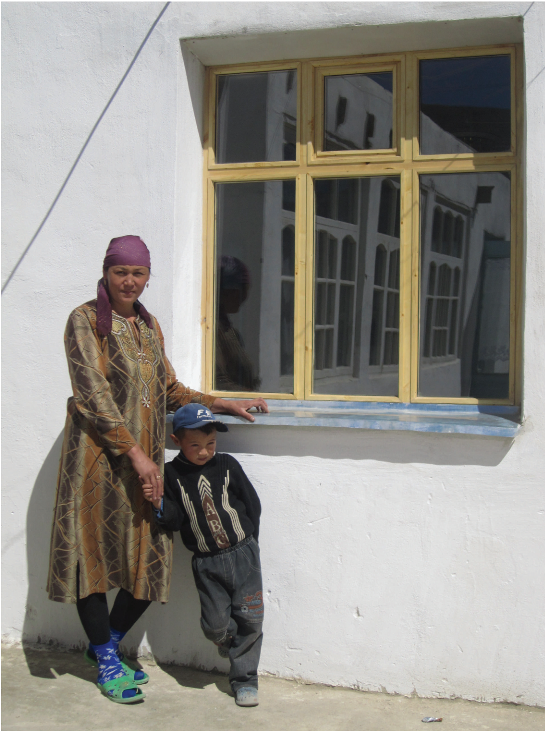
FIGURE 4 The new wooden windows are double glazed and hermetic. In the past, many windows were only single glazed, had broken glass, and were covered with plastic foil during winter to reduce the loss of heat. (Photo by Stefan Salzmann, 2010)
