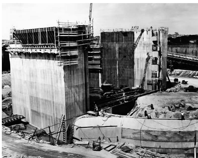
Figure 15. Construction of the sector gatehouse, New Bedford barrier, 1964. The structure in the lower right is a guide for the gate rollers and also contains a tunnel through which the gate operators can walk under the channel (photograph courtesy NAE).
