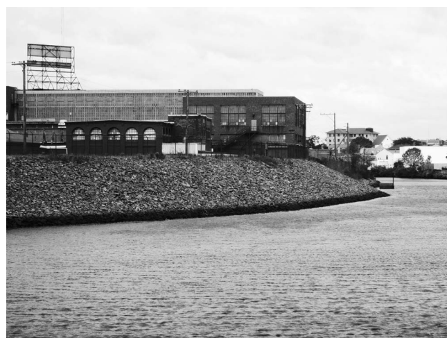
Figure 20. Hurricane surge barrier, west bank of Pawcatuck River, Stonington, Connecticut (photograph by A. Morang, taken from Westerly, Rhode Island).
