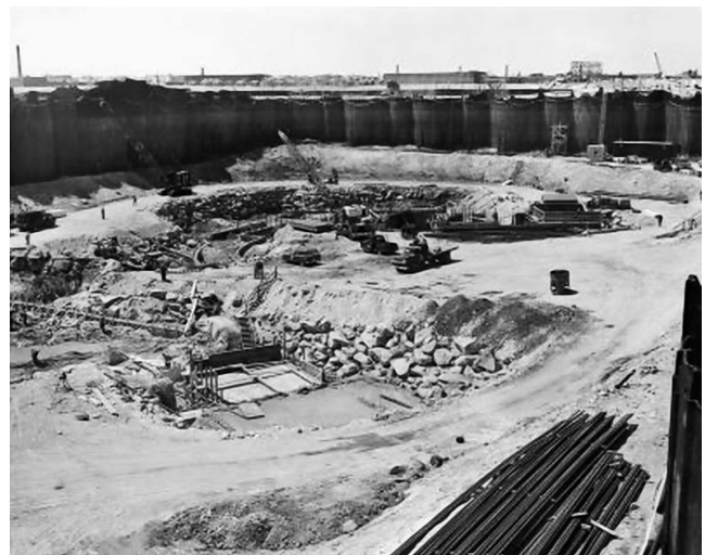
Figure 14. Sector gate foundation work within protective cofferdam, New Bedford harbor, Massachusetts, 5 May 1964 (photograph courtesy NAE).
