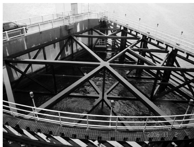
Figure 16. West side sector gate in rest position, New Bedford hurricane barrier, 2 November 2006. The pivot is at the upper center of the photograph, and the ship channel is to the right. Silt builds up in the basin and must be flushed with compressed air. The gate is operated by a 25 hp electric motor (photograph by A. Morang).
