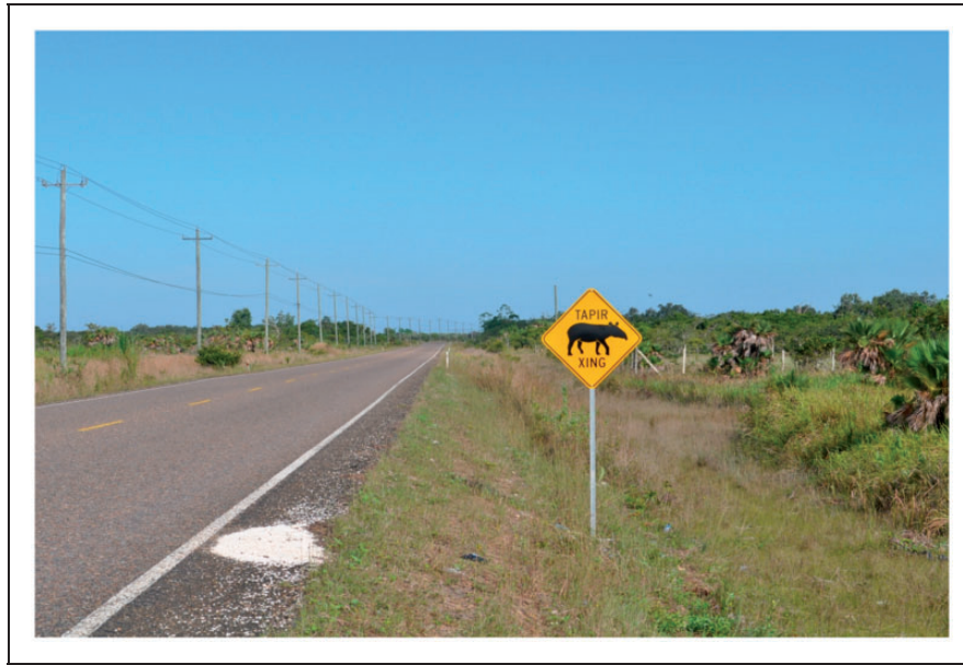
Figure 2. Two sets of reflective wildlife crossing signs were installed at two hot spots identified for tapir-vehicle collisions.
