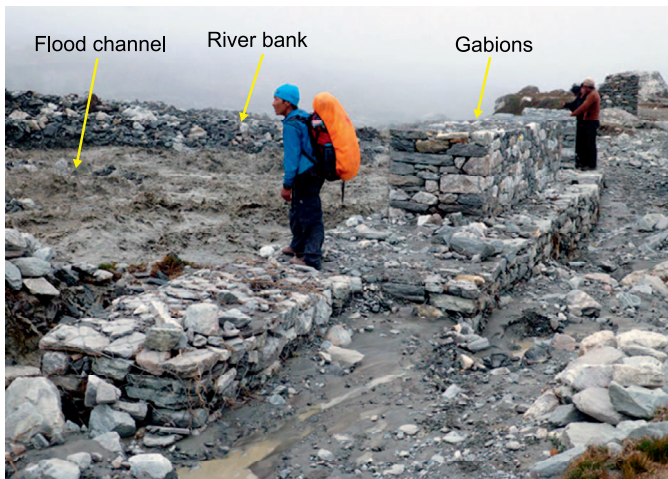
FIGURE 3 Gabions constructed near Chukhung village in 2016, following a threatening englacial flood from the Lhotse glacier in 2015. Local lodge owners credited the gabions with protecting the village during a second flood in 2016. (Photo by Alton C. Byers)
