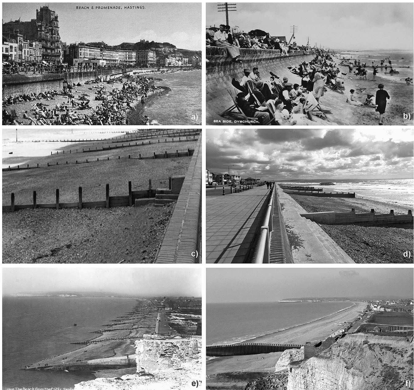
Figure 1. Old and new shore protection structures in U.K. (a) The Hastings seawall in the 1960s (East Sussex Library). (b) Seawall and groynes at Dimchurch, circa 1940s. (East Sussex Library). (c) Towyn, 1960s. (d) Towyn, 2015. (e) Groynes at Seaford, 1912 (East Sussex Library). (f) Seaford, current conditions (East Sussex Library).
