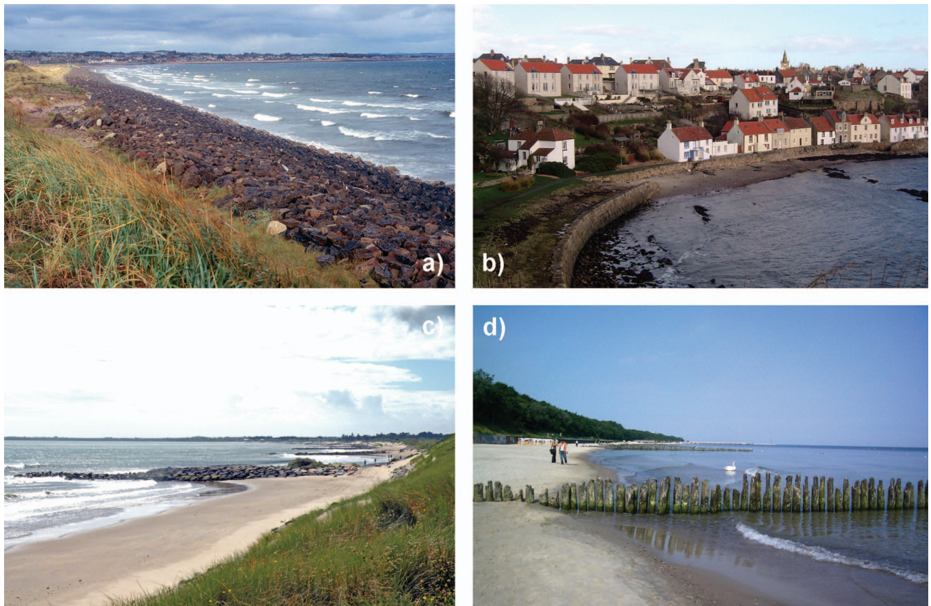
Figure 2. Shore protection structures in use in RCCEA times. (a) 3 km long rubble-mound rock armour revetment, Buddon Ness, Scotland. Built 1992/3 by Ministry of Defence to protect a military training area. Sand/beach interchange is now inhibited causing degraded dunes. Photo by Robert W. Duck. (b) Vertical masonry walls dating back to the 1800s at Pittenweem, Scotland. It has been repaired many times. Photo by Robert W. Duck. (c) Rock groynes (Rosslare, Ireland). (d) Wood permeable groyne (Kotobrzeg, Poland).
