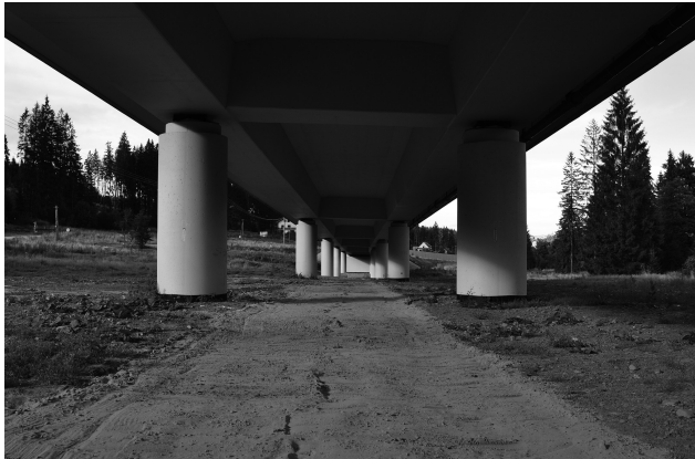
Fig. 2. The wildlife crossing structure underpass near Laliki village on the S69 express road in western Polish Carpathians (photographed by Robert W. Mysłajek).
