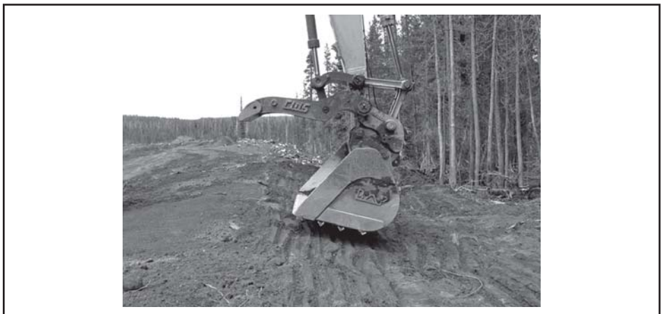
Figure 6. Bucket imprinting is used to press soil into place, but does not compact soils to negatively impact revegetation.
