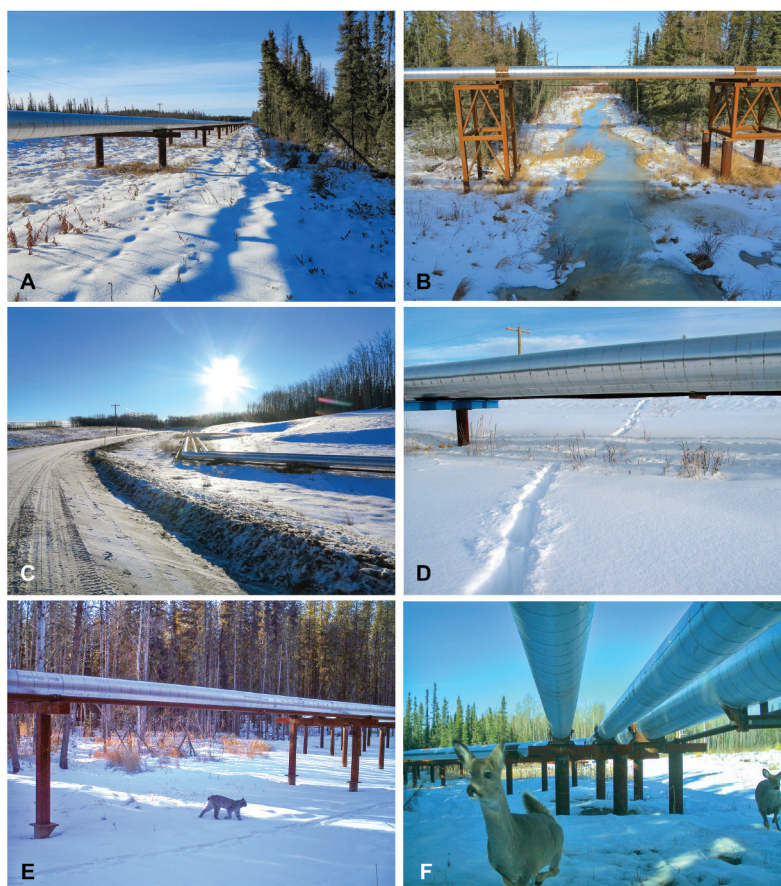
Figure 2. Example photographs showing A) above-ground pipeline paralleling forest; B) above-ground pipeline crossing a riparian area; C) above-ground pipeline paralleling a service road; D) grey wolf ( Canis lupus ) trail under the above-ground pipeline; E) Canada lynx ( Lynx canadensis ) crossing under the above-ground pipeline; and F) white-tailed deer ( Odocoileus virginianus ) crossing under the above-ground pipeline.
