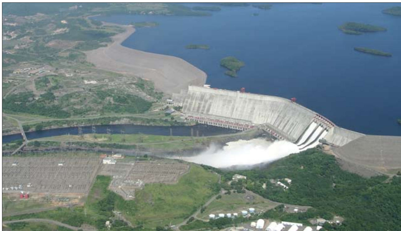
Figure 2.15. Large hydroelectric projects like the Raul Leoni Dam at Gurí on the Caroni River in Venezuela provide subsidized energy for aluminum smelters. Like many dams, it is situated near the mouth of a large river to maximize electrical energy production, which depends on water volume and vertical drop. However, placing the dam at the mouth of the river also isolates fish populations of the entire watershed from the rest of the Orinoco basin (© Daniela Vizcaino/CI).
