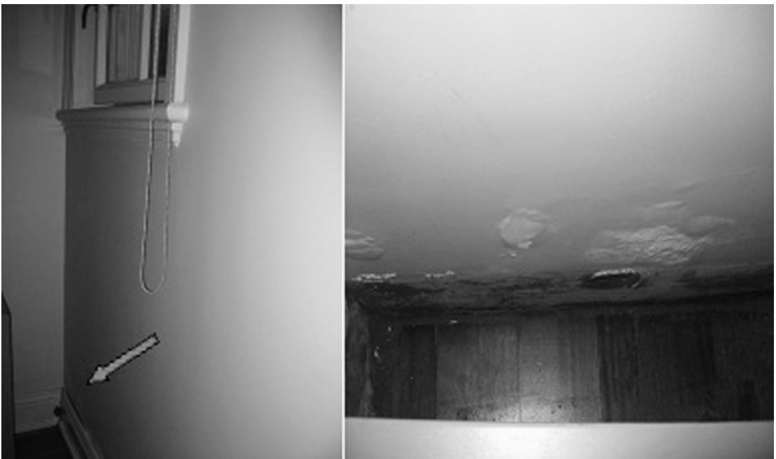
Fig. 3. Effect of high air humidity in basement.
