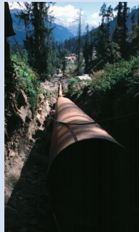
FIGURE 1 Construction of a pipeline in Solang. This steep pipe, with a diameter of 1.1 meters, leads to a 3MW potential power house over a distance of 2 km. (Photo by author)
