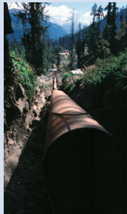
FIGURE 1 Construction of a pipeline in Solang. This steep pipe, with a diameter of 1.1 meters, leads to a 3MW potential power house over a distance of 2 km. (Photo by author)
