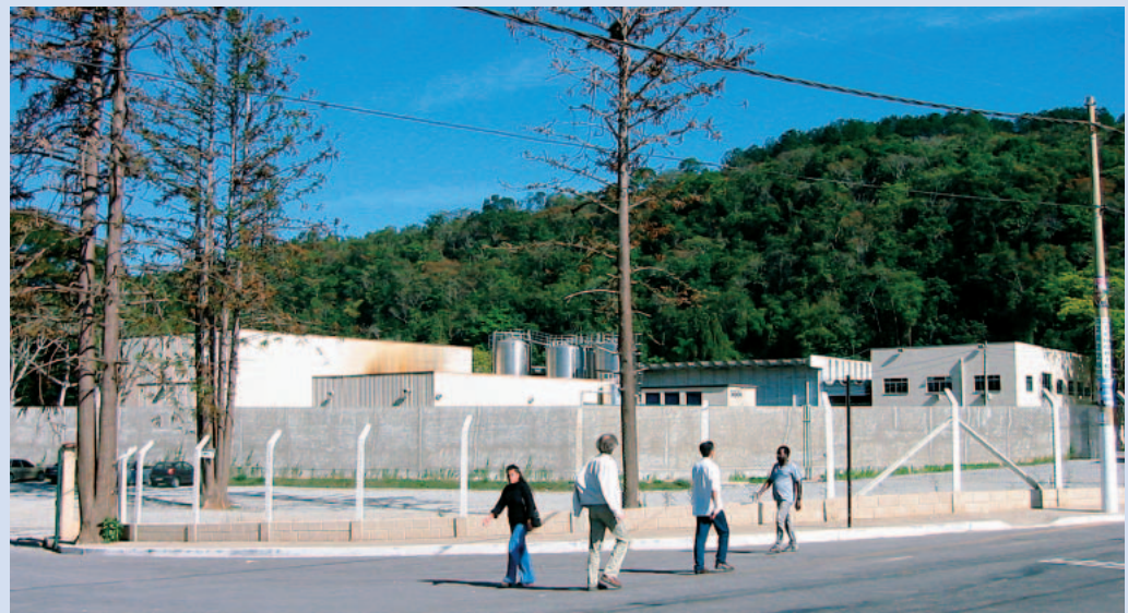
FIGURE 3 The site of the Nestlé/Perrier Pure Life bottling plant. Has water extraction been so intense that trees in the area have perished? (Photo by Stephan Rist)
