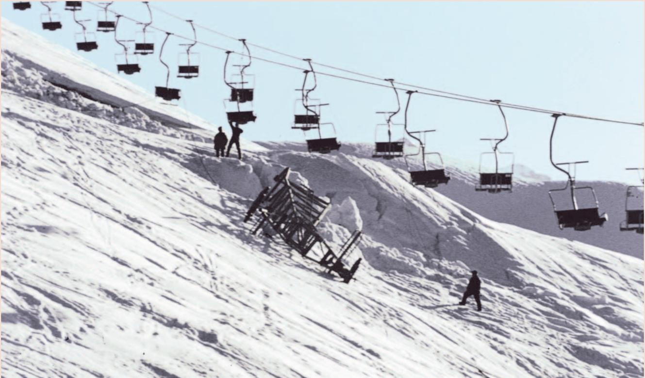
**FIGURE 3** Chair lift pylon damaged by snow pressure on 14 March 1999, in Hasliberg (Canton of Berne, Switzerland). (Photo courtesy of SLF)
