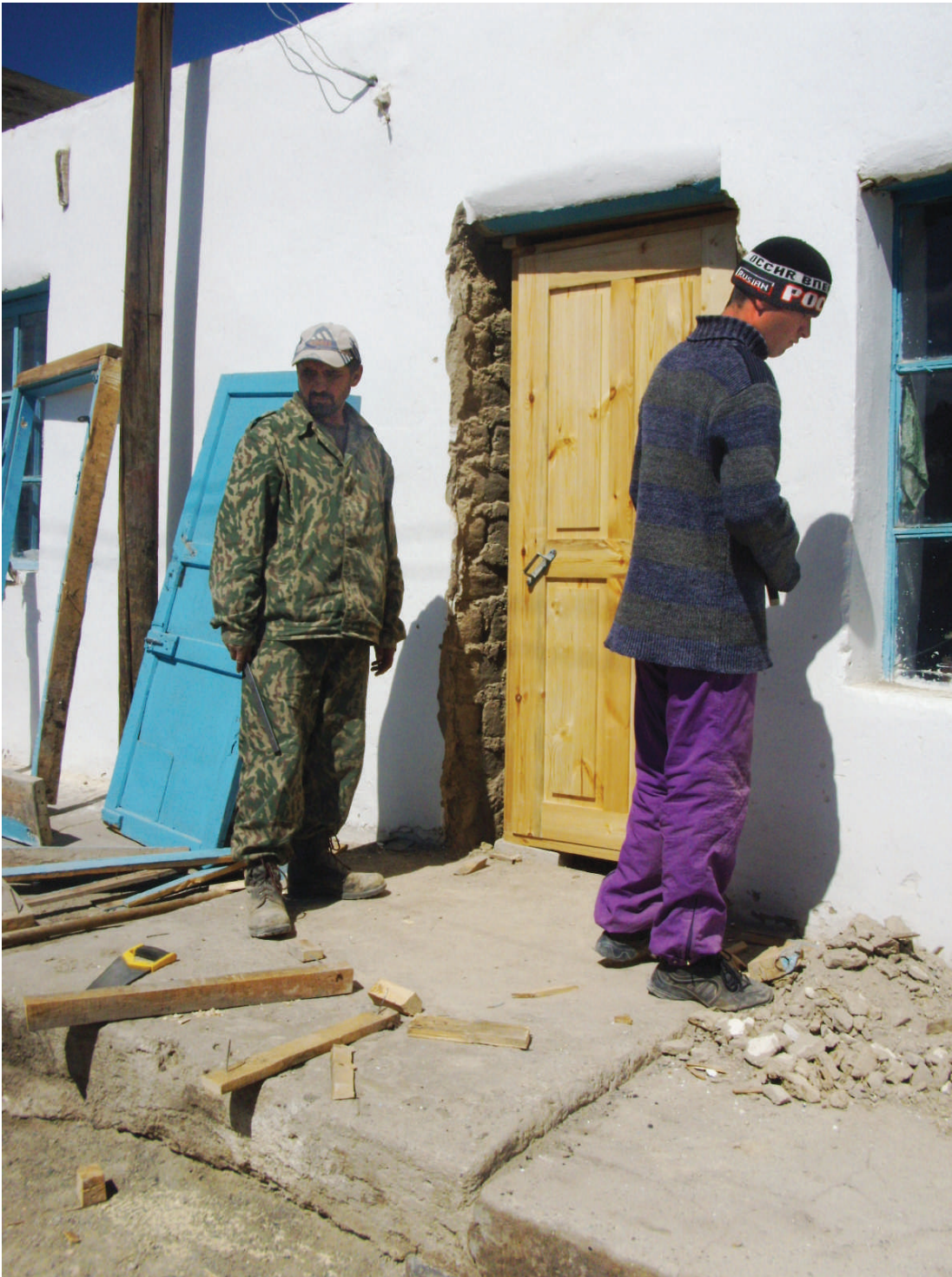
FIGURE 3 Construction workers in Murgab are installing a hermetically closing wooden door produced by carpenters in Khorog. (Photo by Rustam Zevashoev 2010)
