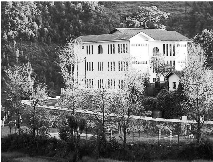
FIGURE 3 Newly created Block Administrative Centres support a cluster of 5 to 6 gram panchayats and have helped strengthen governance and last mile program delivery. (Photo by Sandeep Tambe)
