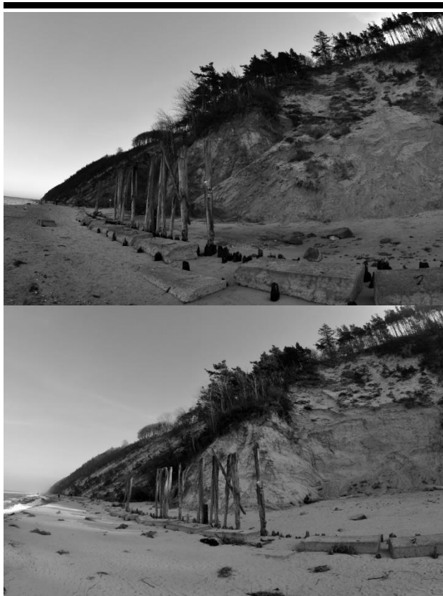
Figure 4. Wolin cliff coast in section I. Situation before (upper image) and after (bottom image) the 4 th January storm.
