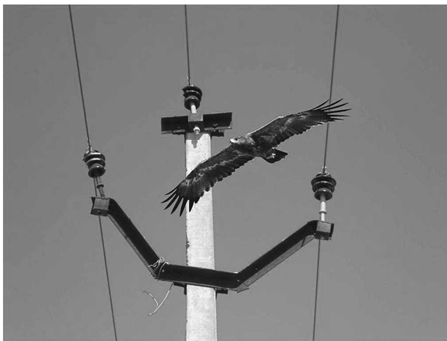
Figure 1. Typical 11-kV concrete pole with a grounded metal cross-arm. A Steppe Eagle ( Aquila nipalensis ), a common raptor in Rajasthan, India, with a wingspan of 165–190 cm, provides a reference for relative size.
