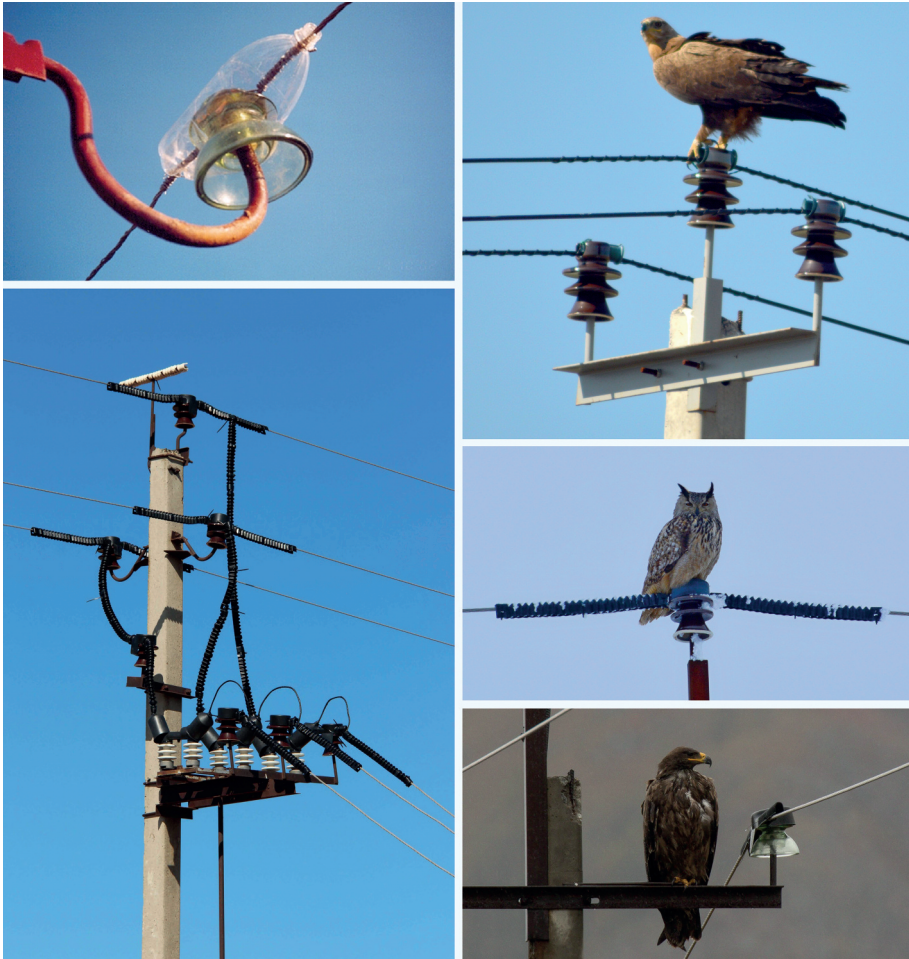
FIG. 6.— Bird Protection Devices (BPDs) designed specifically to fit the 6-10kV electric system in Kazakhstan and southern Russia. Top left: A plastic bottle used before BPDs were available in the region (photo: Adrey Saltykov from Medzhidov et al. , 2005). Top right: a Steppe Eagle Aquila nipalensis perched on insulated wire in Southern Ural, Russia (photo: Igor Karyakin). Centre right: A Eurasian Eagle-Owl Bubo bubo perched on a conductor cover in the Kalmykia, Russia (photo: Gennadiy Erdnenov). Bottom left: BPDs on conductors, jumpers, and equipment on a switch pylon (photo: EcoNIOKR). Bottom right: Steppe Eagle perched adjacent to a conductor fitted with a cover in Altai, Russia (photo: Márton Horváth).
