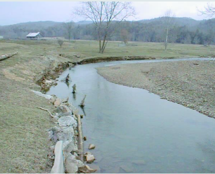
FIGURE 6 Channelizing in the Knapps Creek watershed has been an unsuccessful conventional approach to combating bank erosion. (Photo by Gary Berti)
