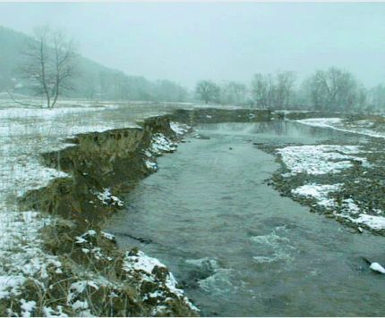
FIGURE 5 Bank erosion along Knapps Creek. (Photo by Gari Berti)
