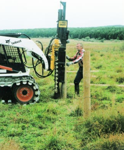
FIGURE 3 Installing fenceposts to protect Bliester Swamp. (Photo by Alton Byers)
