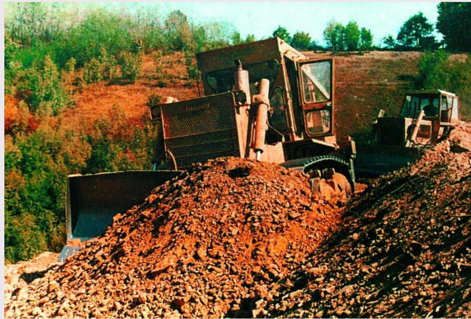
FIGURE 2 The “Feat of the Century”: heavy machinery prepares terraces on the steep slopes of Mt Kukavica. (Photo courtesy of Porecje Company)
