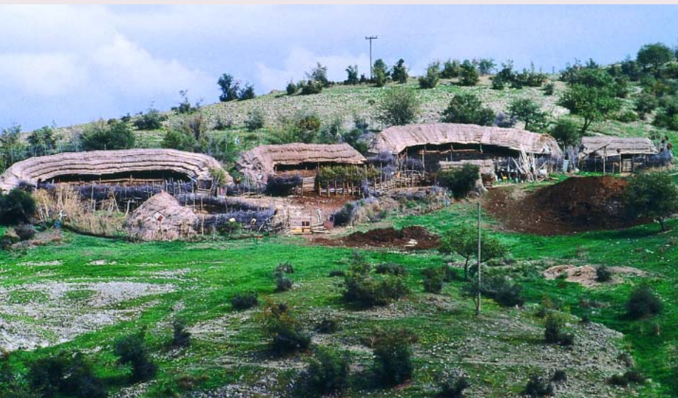
FIGURE 2 Traditional Sarakatsaniko sheepfolds are built in a semicircular shape with southern exposure to receive sunlight and protection from the north winds. These structures are being used again as a result of the revival of the area. (Photo courtesy of WWF Greece, Kostas Pistolas)
