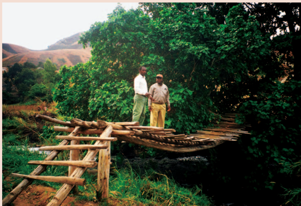
FIGURE 3 The Lubigwa pedestrian bridge, built using traditional methods pre-dating the new suspension technology. (Photo by Mr. Kanyunyu, ITECO)
