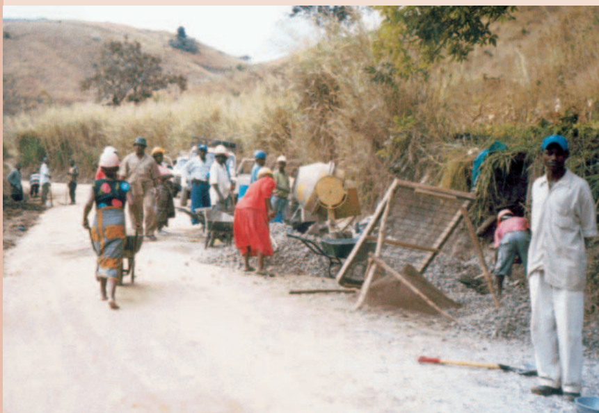
FIGURE 1 Local people rehabilitating the Mlali to Mgeta road in the Uluguru mountains. (Photo by Mr. Karumuna, ITECO)
