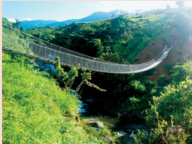
FIGURE 2 The new Kipondwa pedestrian bridge. (Photo by Mr. Kanyunyu, ITECO)
