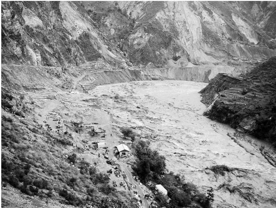
FIGURE 1 Neelum River and road near quarry north of Muzaffarabad. (Photo by Rauf Qureshi, 2010)
