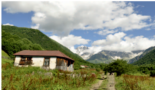
FIGURE 5 Abandoned house in the village of Gona in the high-elevation mountainous zone. This remote village was completely abandoned already in 1989; see Figure 4 for its location. (Photo by G. Dvalashvili)
