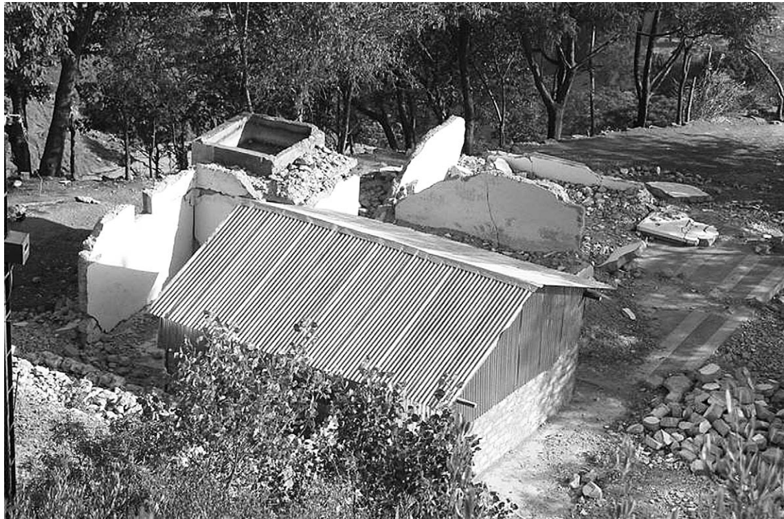
FIGURE 2 The government recommended-rebuilding scheme incorporates the use of a wood frame with 90–120 centimeters of brick or concrete on the lower walls and corrugated galvanized iron (CGI) sheets for upper walls and roofs. Among those interviewed in Pakistani administered Kashmir, 80% felt that this was the best technique for rebuilding. (Photo by J.P. Hamilton, June 2006)
