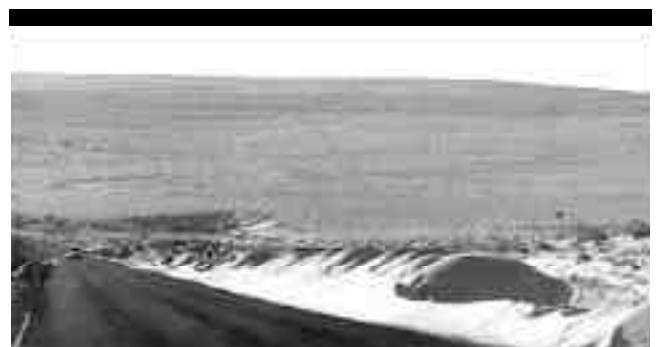
Figure 5. The road is an obstacle to sand transport although in some places sand overpasses it. Sediment transport is from right to left.
