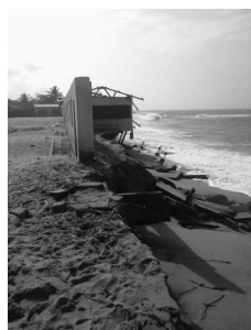
Figure 4. Collapsed school building in Fuvemeh community, which illustrates the effect of coastal erosion on vulnerable delta communities (taken June 2016).
