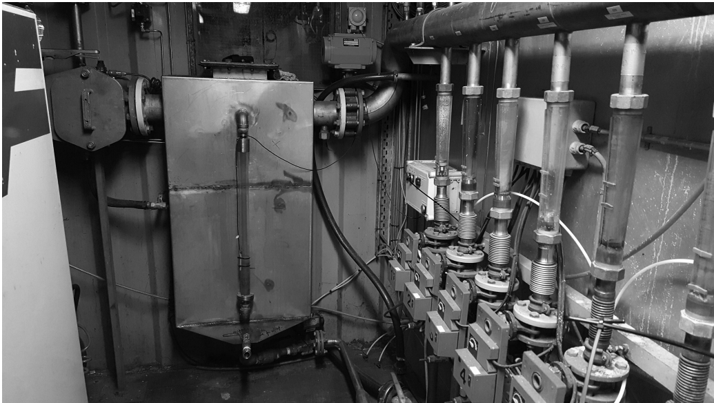
Figure 3. Milking apparatus to separate water and methane. (Photo by authors)
