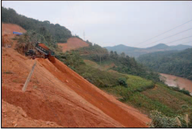
Figure 5. Road construction and disposal of debris over the edge of the road and the impact on the local river; the river is the same color as the earth being dumped. Lang Son Province, Vietnam. Photograph by Arthur Bogan. November 11, 2012.
