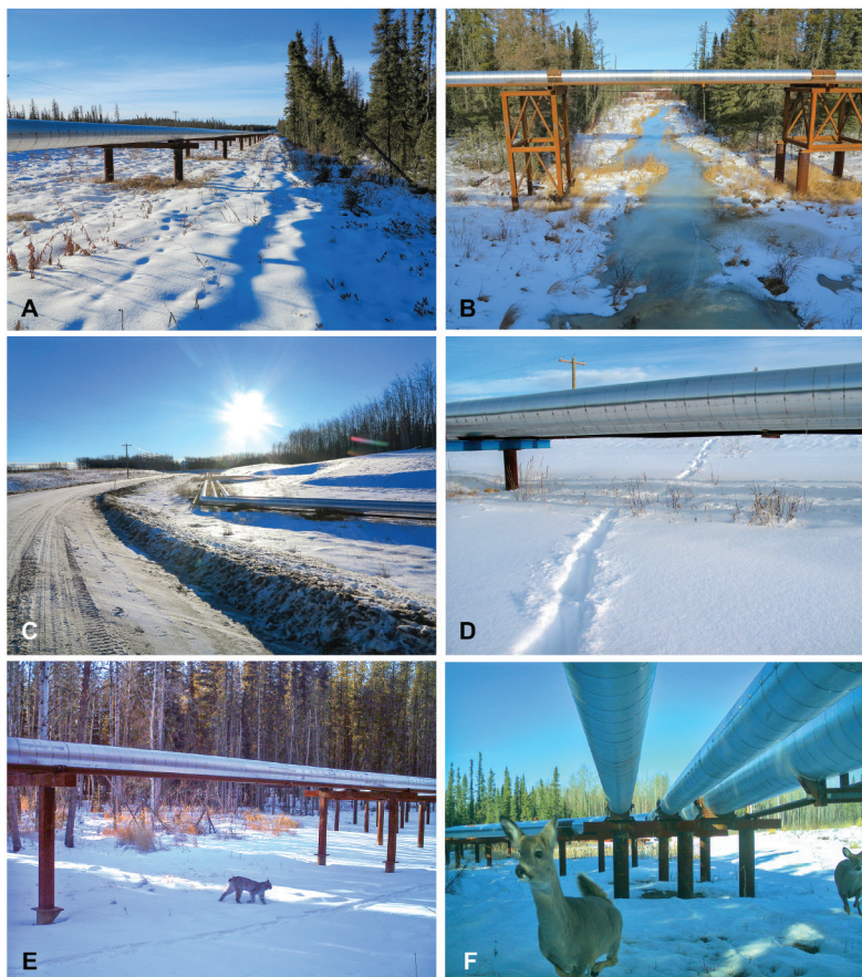
Figure 2. Example photographs showing A) above-ground pipeline paralleling forest; B) above-ground pipeline crossing a riparian area; C) above-ground pipeline paralleling a service road; D) grey wolf ( Canis lupus ) trail under the above-ground pipeline; E) Canada lynx ( Lynx canadensis ) crossing under the above-ground pipeline; and F) white-tailed deer ( Odocoileus virginianus ) crossing under the above-ground pipeline.
