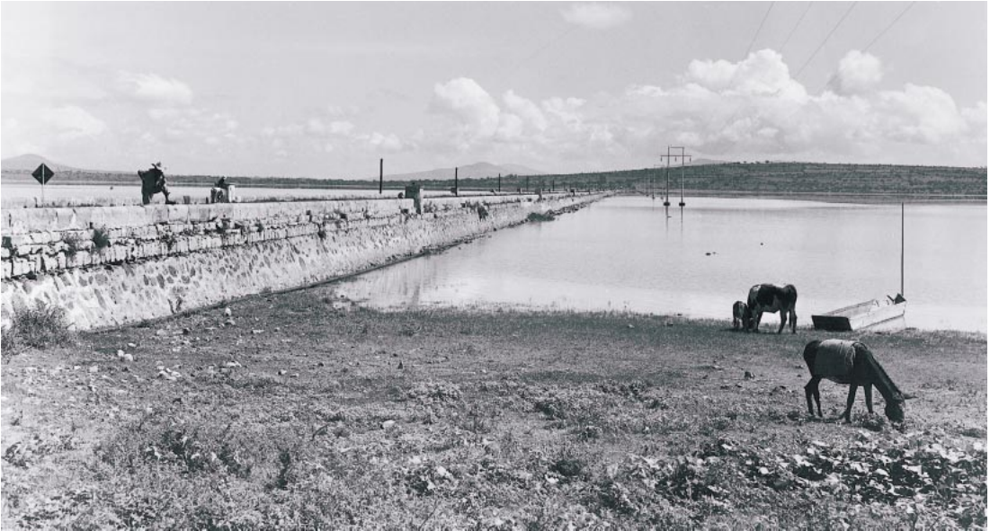
Fig. 2. Lago de Cuitzeo, Michoacán. South shore and southern end of the 19th-century causeway across the lake.
