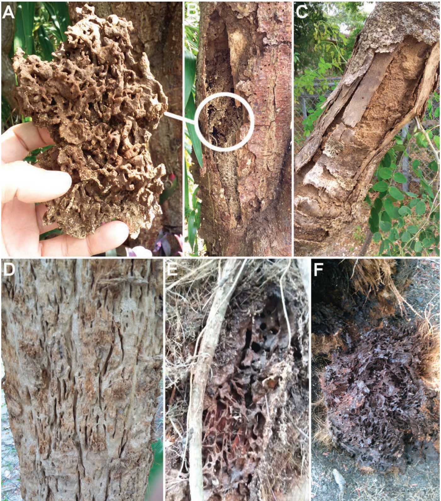
Fig. 2. Feeding damage from Coptotermes gestroi on various tree species. (A) Carton material extracted from (B) a dead gumbo-limbo tree ( Bursera simaruba ); this tree was still alive less than 1 yr before the picture was taken. (C) Termite feeding damage on a Senna surattensis , still alive, but having lost most of its branches. (D) Old scars from feeding damage of C. gestroi on a live sabal palm ( Sabal palmetto ). (E) Active infestation and carton material in the trunk of a live sabal palm. (F) Carton material in the heart of a dead pindo palm ( Butia capitata ).
