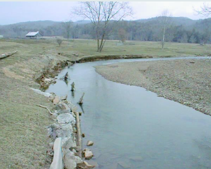
FIGURE 6 Channelizing in the Knapps Creek watershed has been an unsuccessful conventional approach to combating bank erosion. (Photo by Gary Berti)
