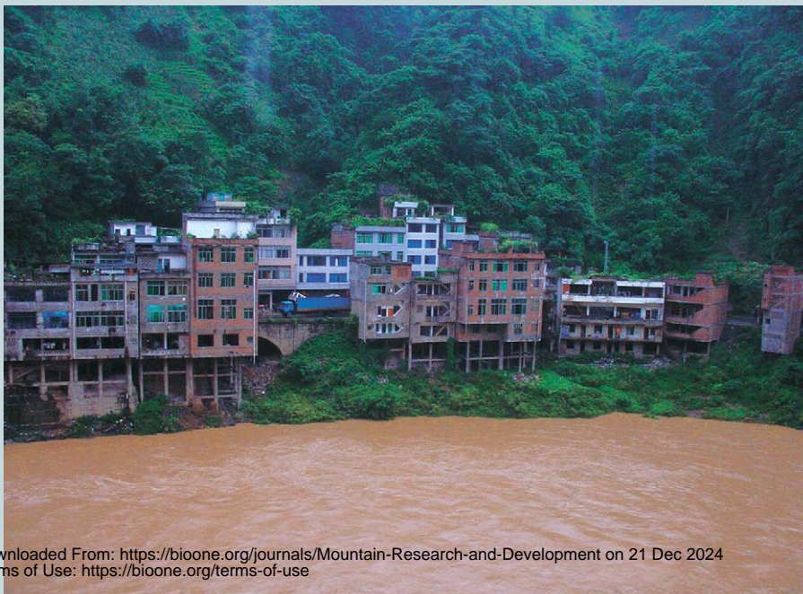
FIGURE 2 Buildings on concrete stilts show the extreme scarcity of flat land suitable for construction in the densely populated Zhaotong City area. (Photo by Zhang Baiping)
