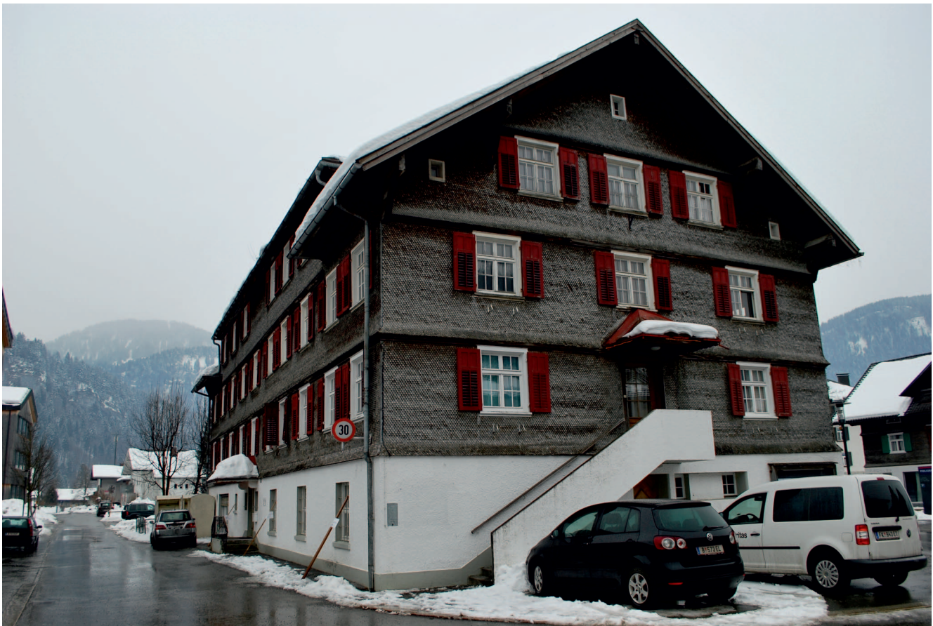
FIGURE 3 The refugee home in the town center of Bezau. (Photo by Elke Kager)
