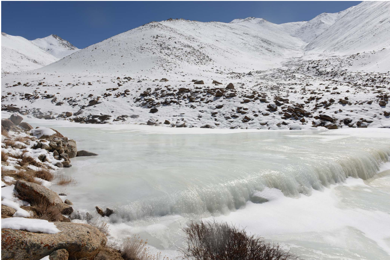
FIGURE 7 Efficient ice accumulation in a cascade-type reservoir in the Igloo catchment. The entire riverbed is filled with ice, and the cascades are completely iced over. (Photo by Marcus Nüsser, 25 February 2014)
