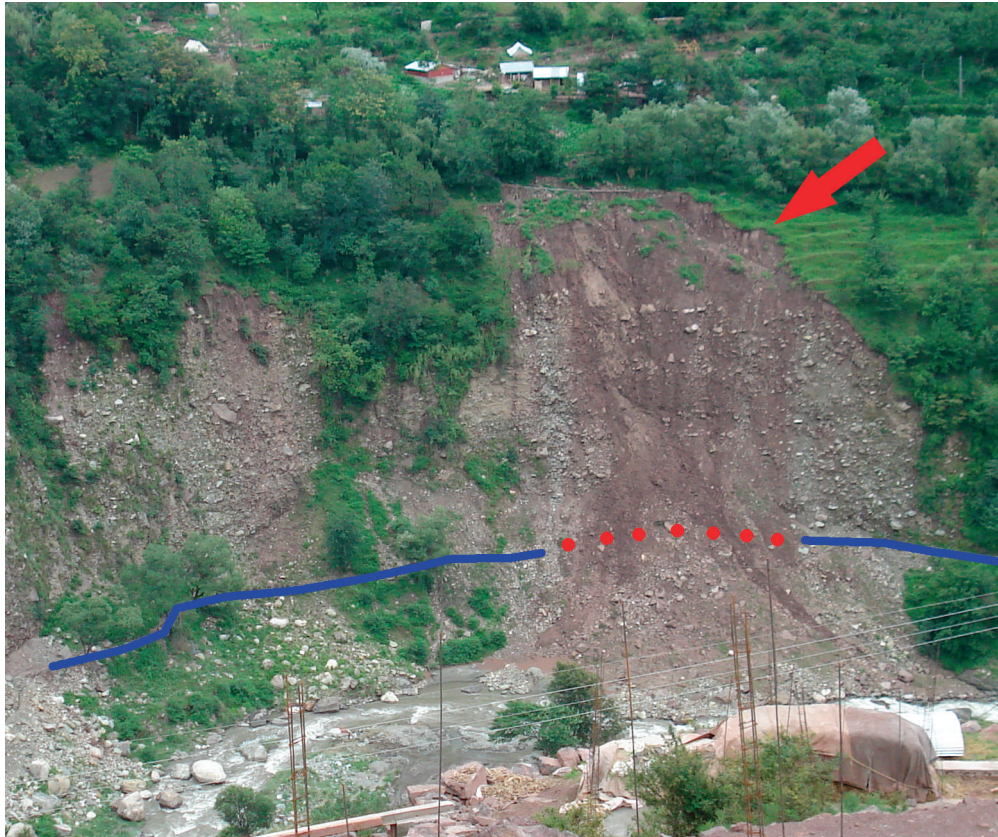
FIGURE 6 Kathai irrigation canal (blue line); most critical section for rehabilitation (red dots) with highly unstable slope above (arrow). (Photo by Markus Zimmermann, 3 July 2007)
