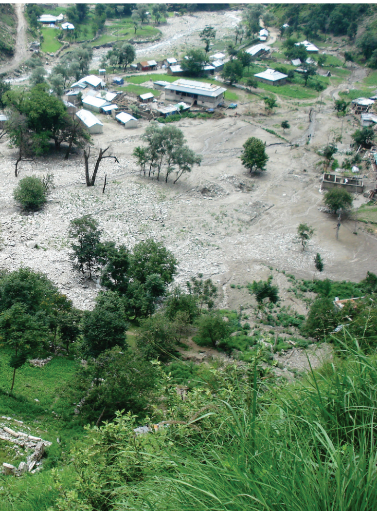
FIGURE 2 Debris flow in March 2007 caused further damage to shelters built after the earthquake at Nardajian (upper valley). (Photo by Markus Zimmermann, 15 July 2007)
