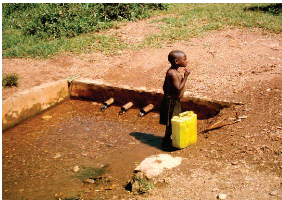
FIGURE 3 Poor maintenance: the immediate surroundings of this protected spring are not maintained. This affects both water quality and yield. (Photo courtesy of Africare, Ntungamo, by Stephen Magume)
