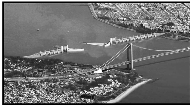
Figure 4. Conceptual design of a storm surge barrier across the Narrows. (Jansen and Dircke, 2009.)
