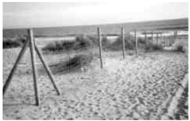
Figure 15. Dune fencing and revegetation in Isla Cristina beach (Huelva, Spain)
