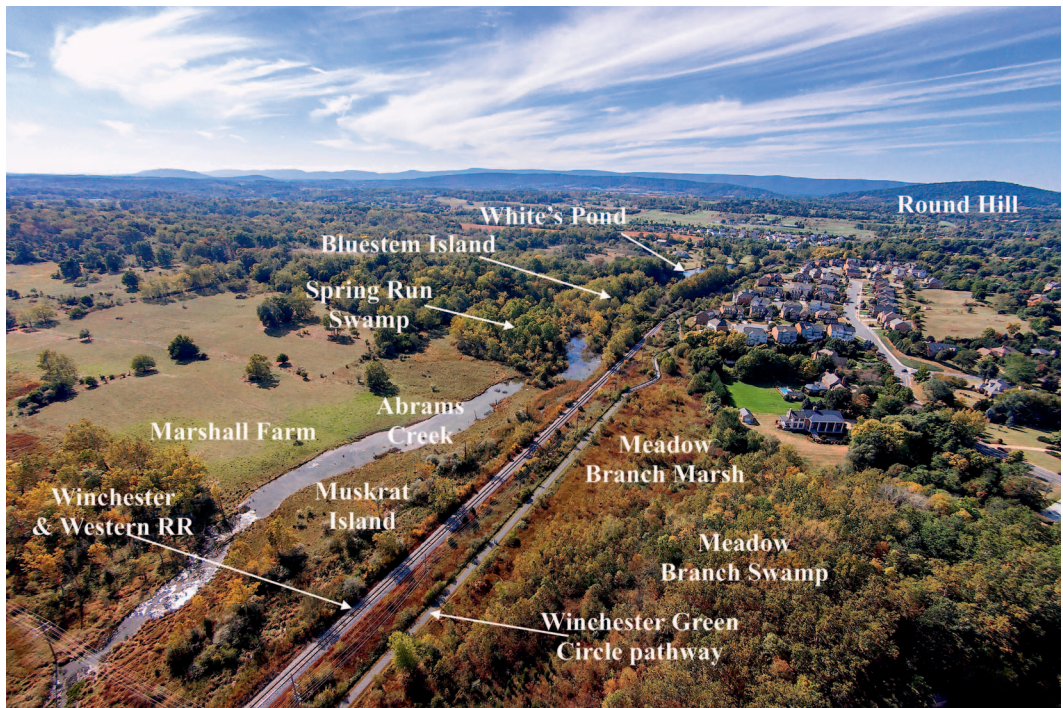
Figure 1. Abrams Creek Wetlands, adjacent land uses, and physiographic setting looking west across the Shenandoah Valley to the Allegheny Mountains. Boundary between Frederick County (left) and Winchester City (right) follows the railroad tracks. Headwaters of Abrams Creek are on Round Hill. Photo by Shaun Galang, Cedarmeade Studios.
