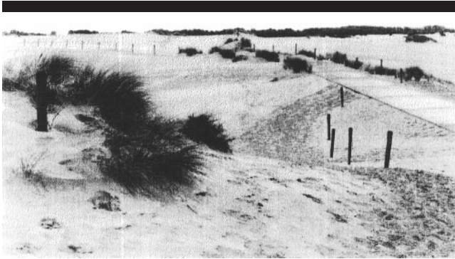
Figure 41. Entrance channels provided for the sea into the dunes where once armored seawalls had toe protection. Photograph courtesy Flemish daily from Ghent; Belgium “Het Volk”.
