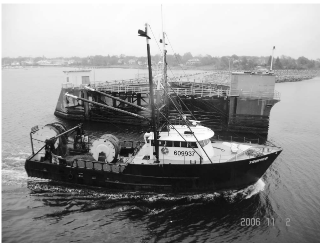
Figure 12. New Bedford hurricane barrier with gate open to allow passage of fishing boat, 2 November 2006 (photograph by A. Morang).
