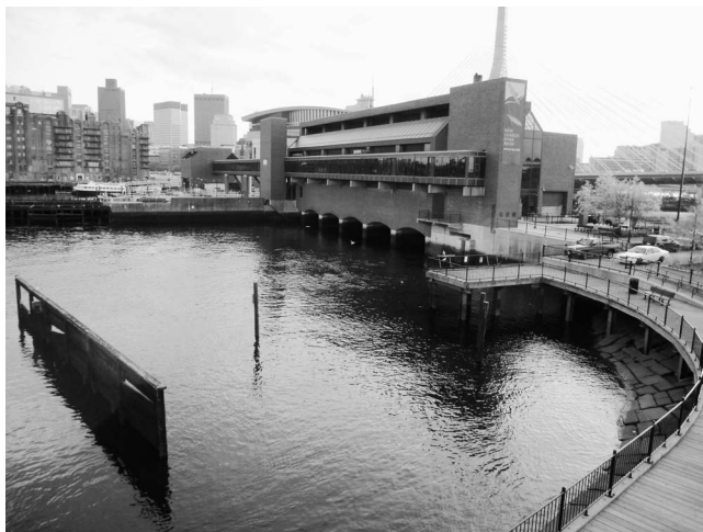
Figure 25. Charles River Dam from Charlestown Bridge (Route 99), view looking south, 1 November 2006. The brick structure contains the pumps. The water in the foreground is the harbor side and is tidal. Downtown Boston is in the distance (photograph by A. Morang).
