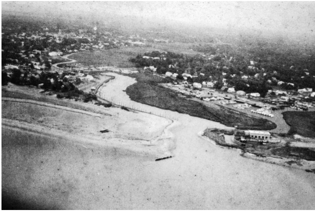
Figure 29. Bayshore pump station at Keansburg, New Jersey, 23 June 1972, 0955 h (photograph courtesy NAN). Levees and floodgate were under construction. The beach to the left had recently been nourished.
