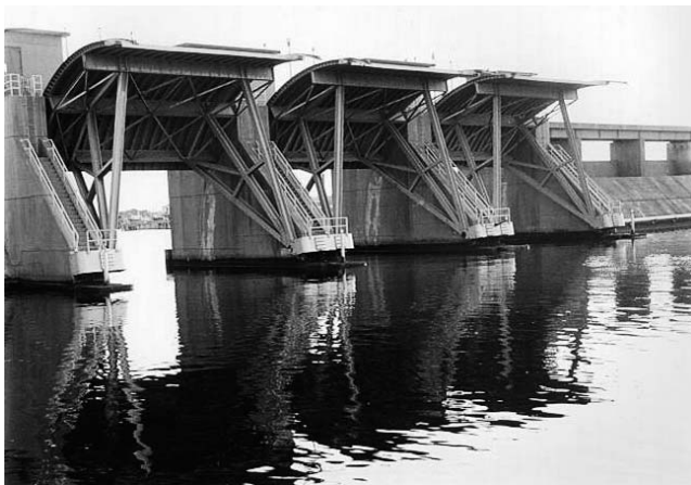
Figure 7. View of the Fox Point tainter gates from the Providence River (north side of the barrier; undated photograph from City of Providence).
