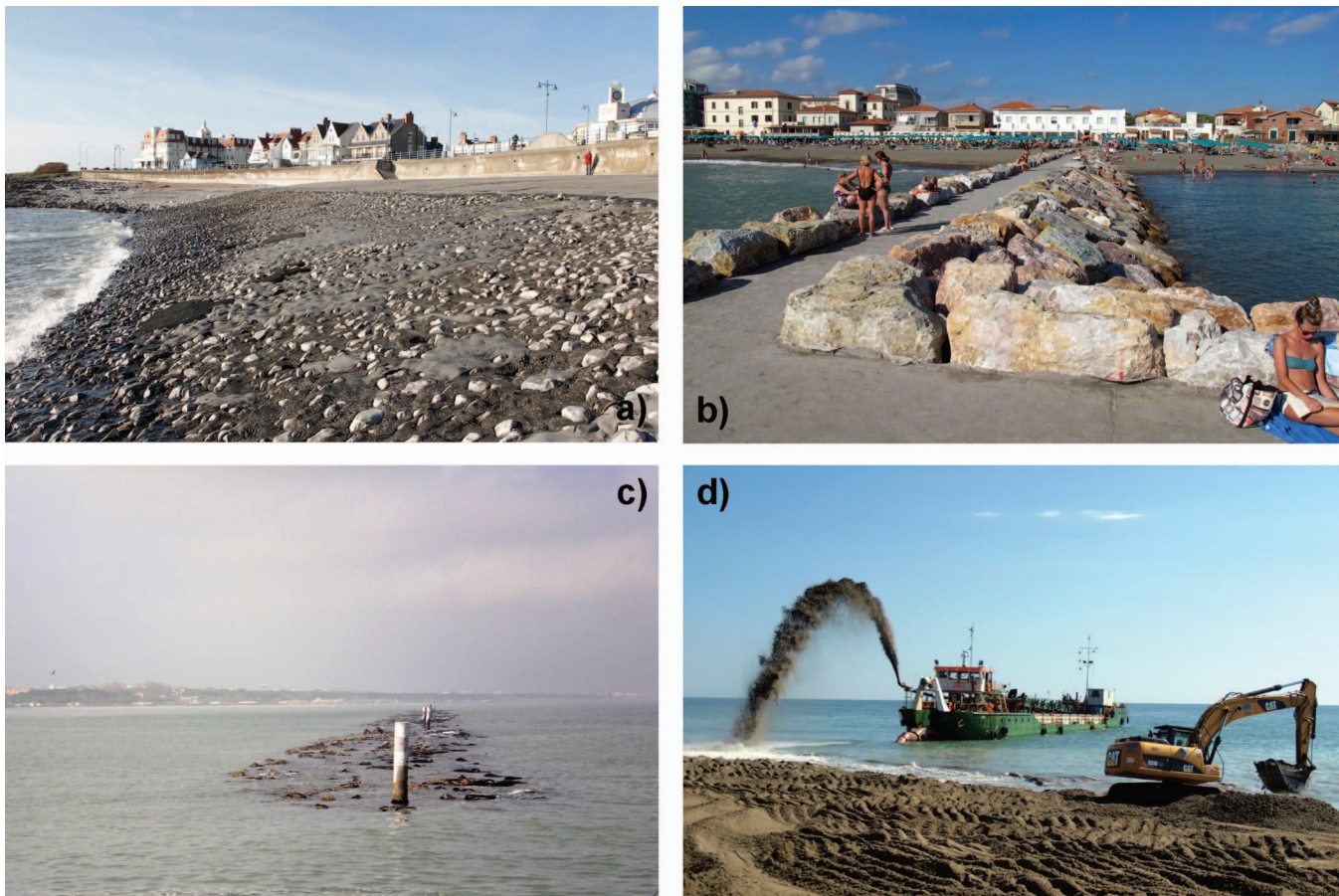
Figure 3. Shore protection projects in use today. (a) Seawall and tar macadam ramp (Porthcawl, Wales). (b) Groyne with a crest walkway (Cecina, Italy). (c) Low-crested breakwaters (Emilia-Romagna coast, Italy). (d) Beach nourishment with “rainbowing” (Tuscany coast, Italy).
