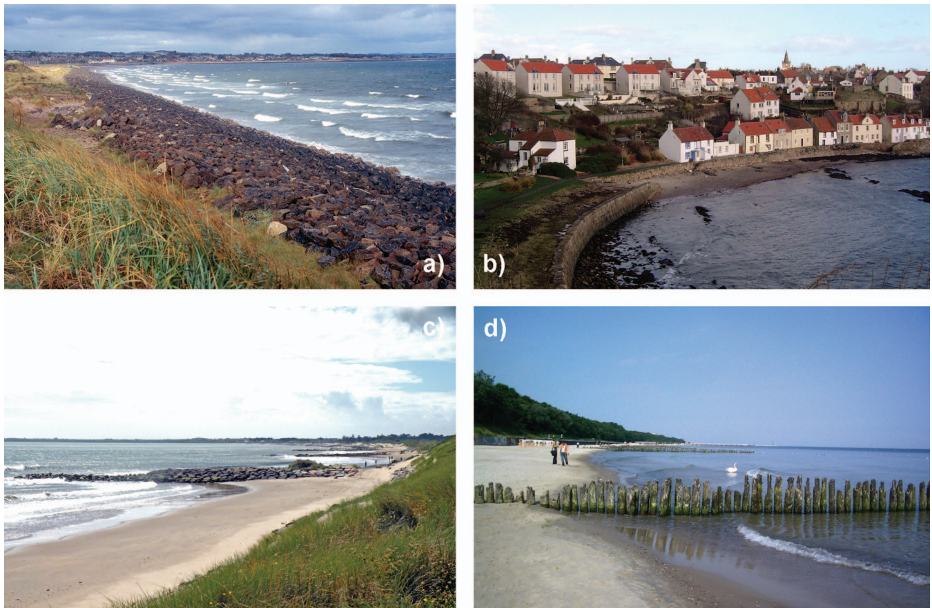
Figure 2. Shore protection structures in use in RCCEA times. (a) 3 km long rubble-mound rock armour revetment, Buddon Ness, Scotland. Built 1992/3 by Ministry of Defence to protect a military training area. Sand/beach interchange is now inhibited causing degraded dunes. Photo by Robert W. Duck. (b) Vertical masonry walls dating back to the 1800s at Pittenweem, Scotland. It has been repaired many times. Photo by Robert W. Duck. (c) Rock groynes (Rosslare, Ireland). (d) Wood permeable groyne (Kołobrzeg, Poland).
